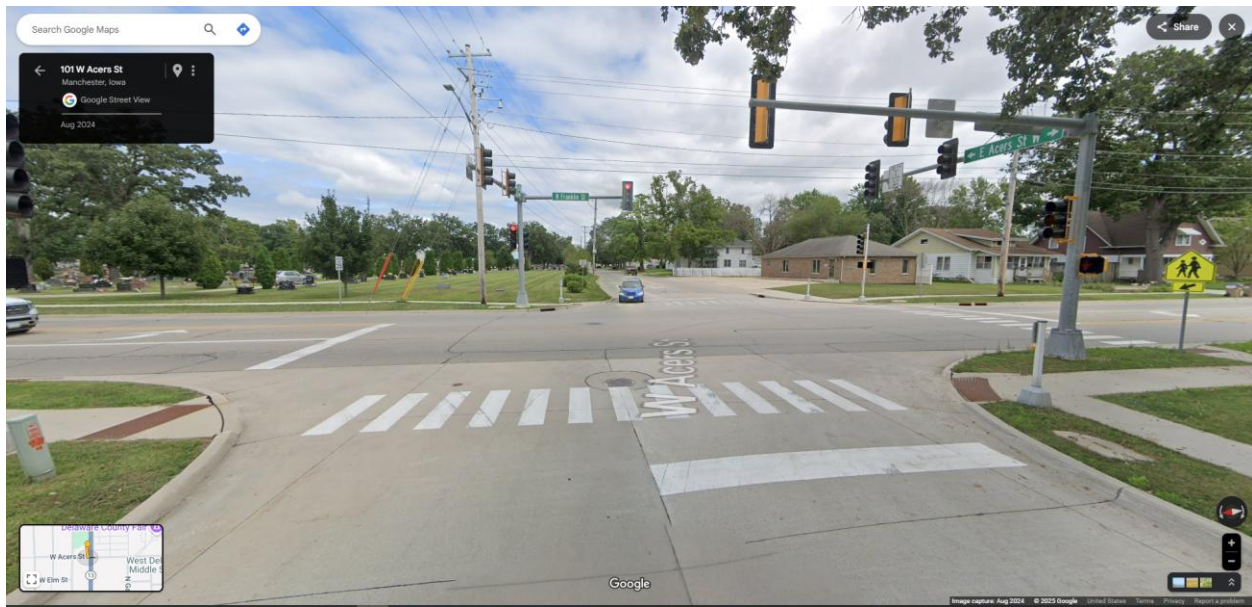
Figure 47: Intersection of N Franklin Street (Iowa 13) and W Acres Street (Image Source: Google )
